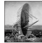
150 ft. diameter dish for radar and communications Stanford University
